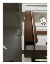
Figure 7: A close up of the mezzanine floor in the Turkish Historical Society. The noncontinuity of the column and the extruded abstracted column head are visible on the left of the wood bookshelf. Source: Photograph by the author.
